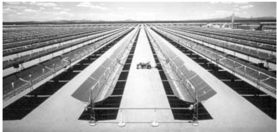
Fig. 9.4.5 - An array of mirrors can concentrate the sun's light onto a black tube containing water. The sunlight striking each mirror is redirected toward the water-filled tube. Here the mirrors form a parabolic arc and the tube rests at the focus of the parabola.
