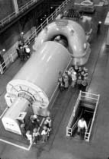
Fig. 9.4.4 - A high-pressure steam turbine drives this electric generator, producing roughly 100 MW of electric power.
