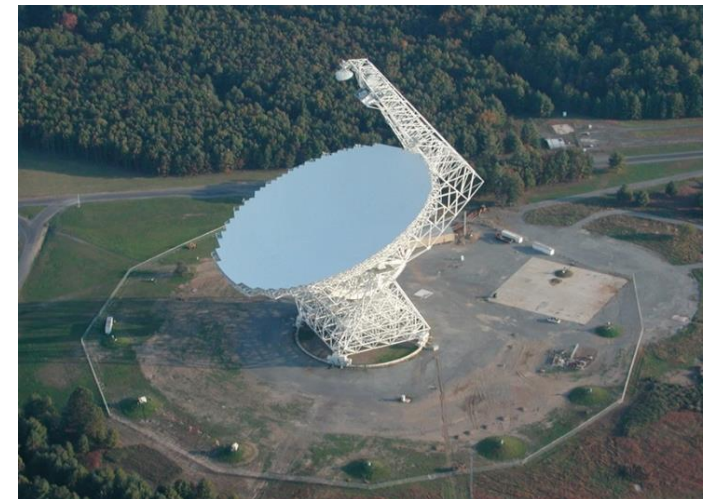
Robert C. Byrd 100 m Green Bank Telescope (GBT) World's largest fully steerable single dish radio telescope
