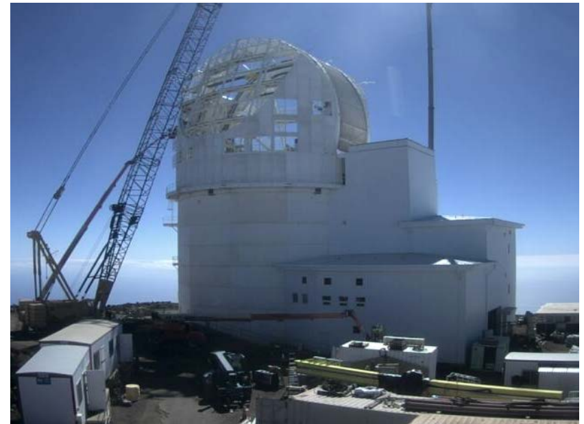
Telescope enclosure assembly underway at the DKIST site on Haleakala, Maui, HI, November 2015. Credit: DKIST project web camera.
